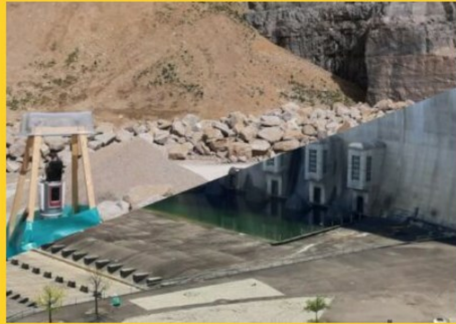
Surface Survey Scan – monitoring
